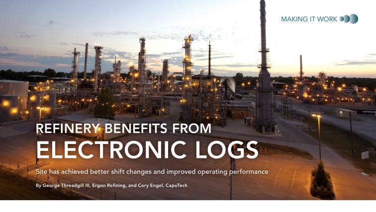
**ERGON REFINING,** Inc. (ERI) operates a 26,500-bbl/d facility in Vicksburg, Miss., that is the world's largest producer of naphthenic specialty oils. The site includes two hydrotreaters, atmospheric and vacuum distillation towers, three hydrogen gas plants, a sulfur recovery unit and a propane deasphalting unit.
